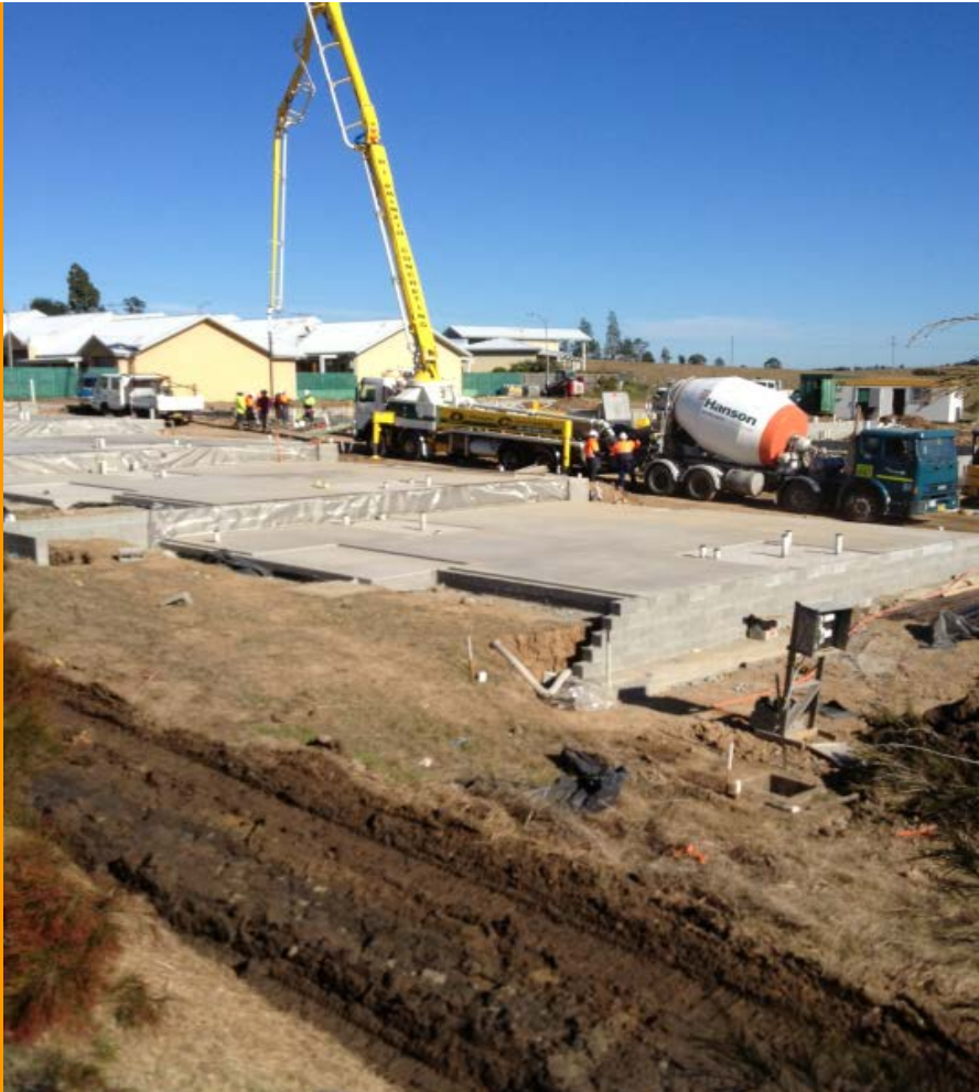
Construction underway for Stage 2 development at Settlers Ridge Estate, Maitland NSW
