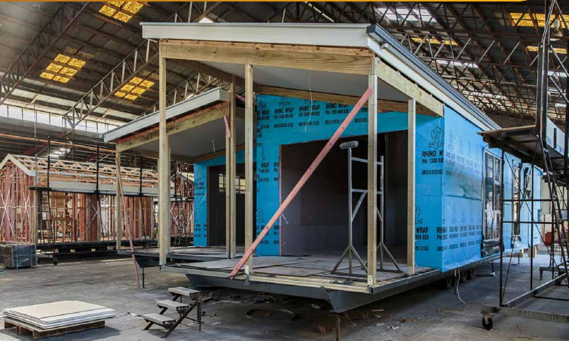
Ingenia home under construction for Stoney Creek
