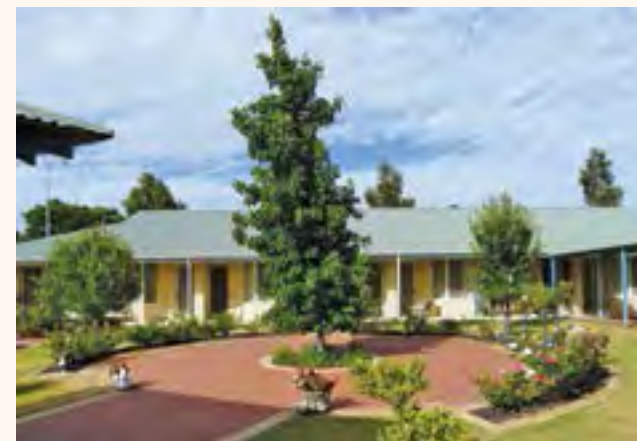
Seville Grove Gardens, Seville Grove, WA
