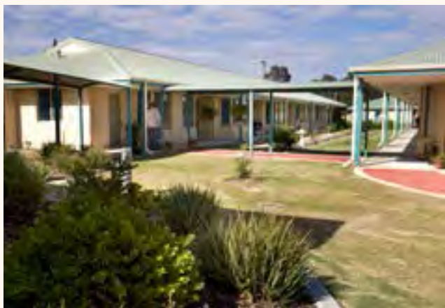
Peel River Gardens, North Tamworth, NSW
