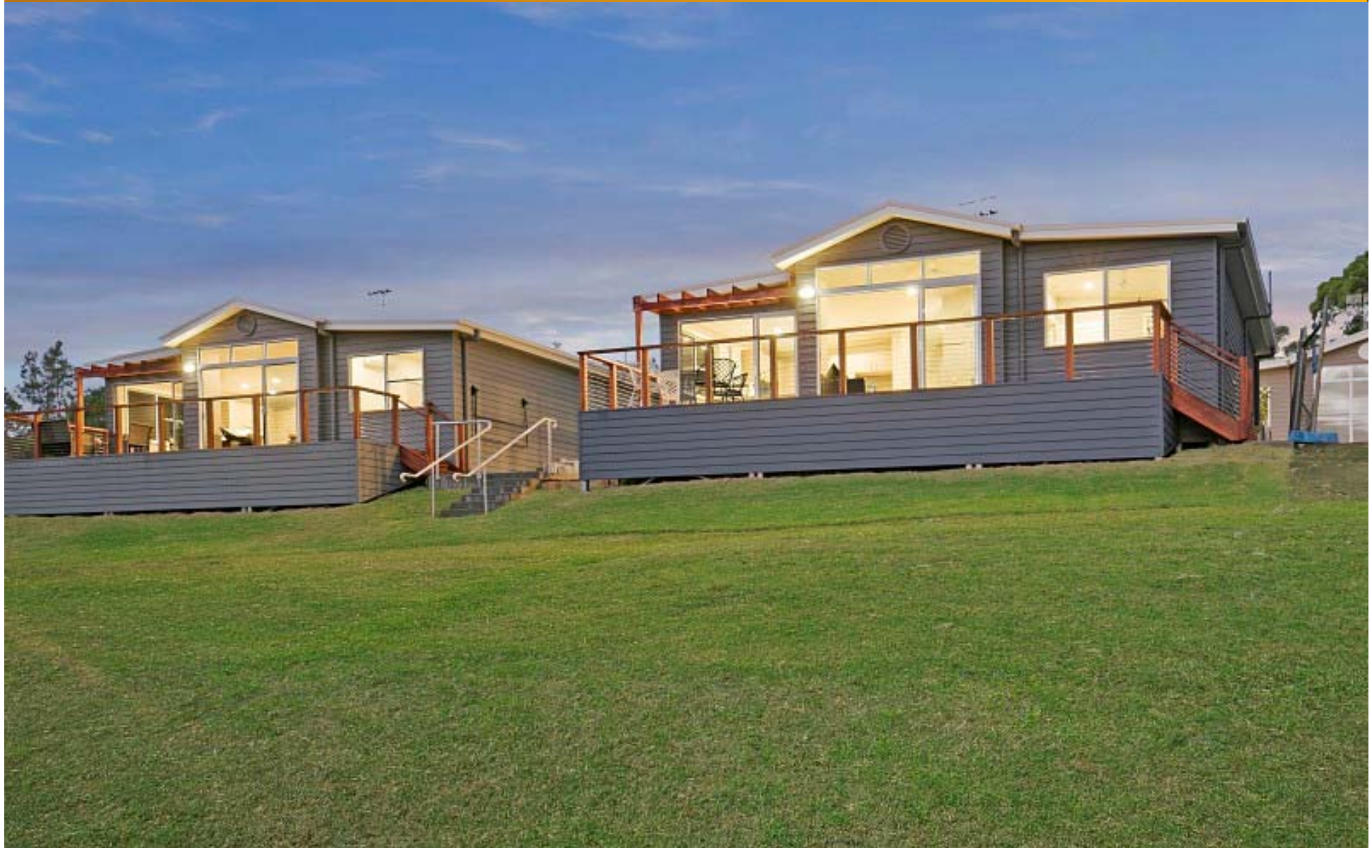
New homes, Chain Valley Bay, NSW
