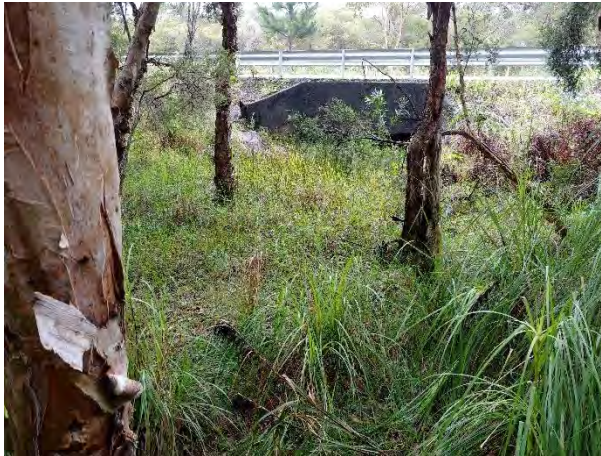
Plate 1: VMA 1, in the west facing culvert
